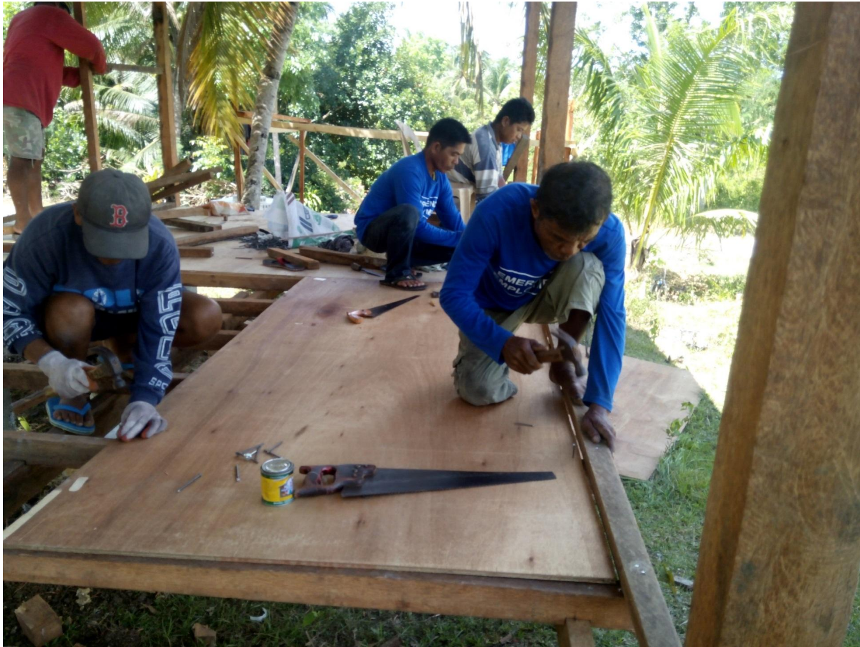
Construct semi-permanent shelters.
