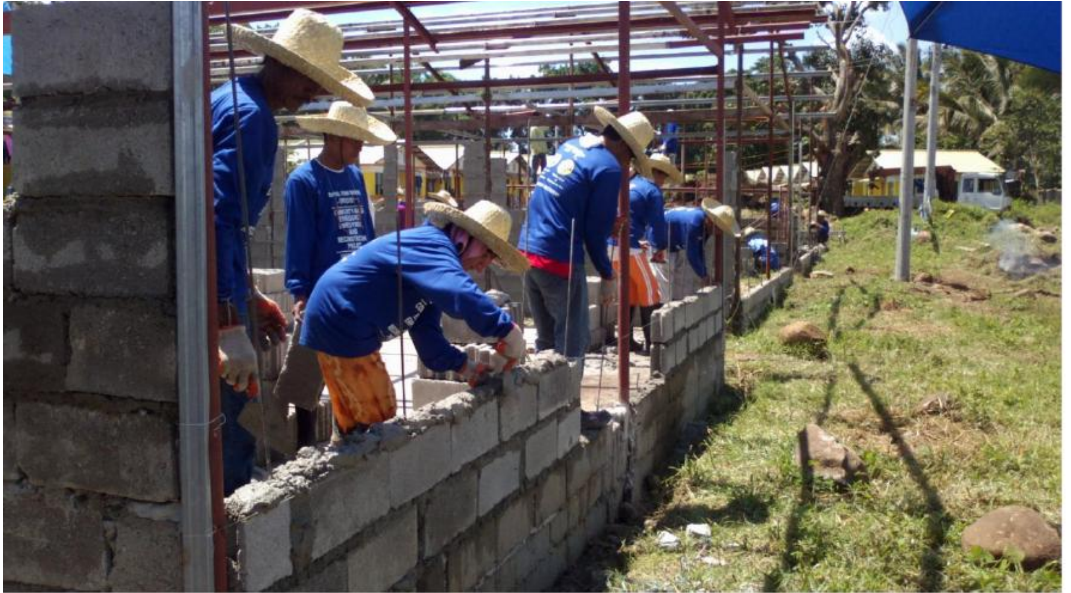
Trained on masonry for the construction of permanent shelters.
