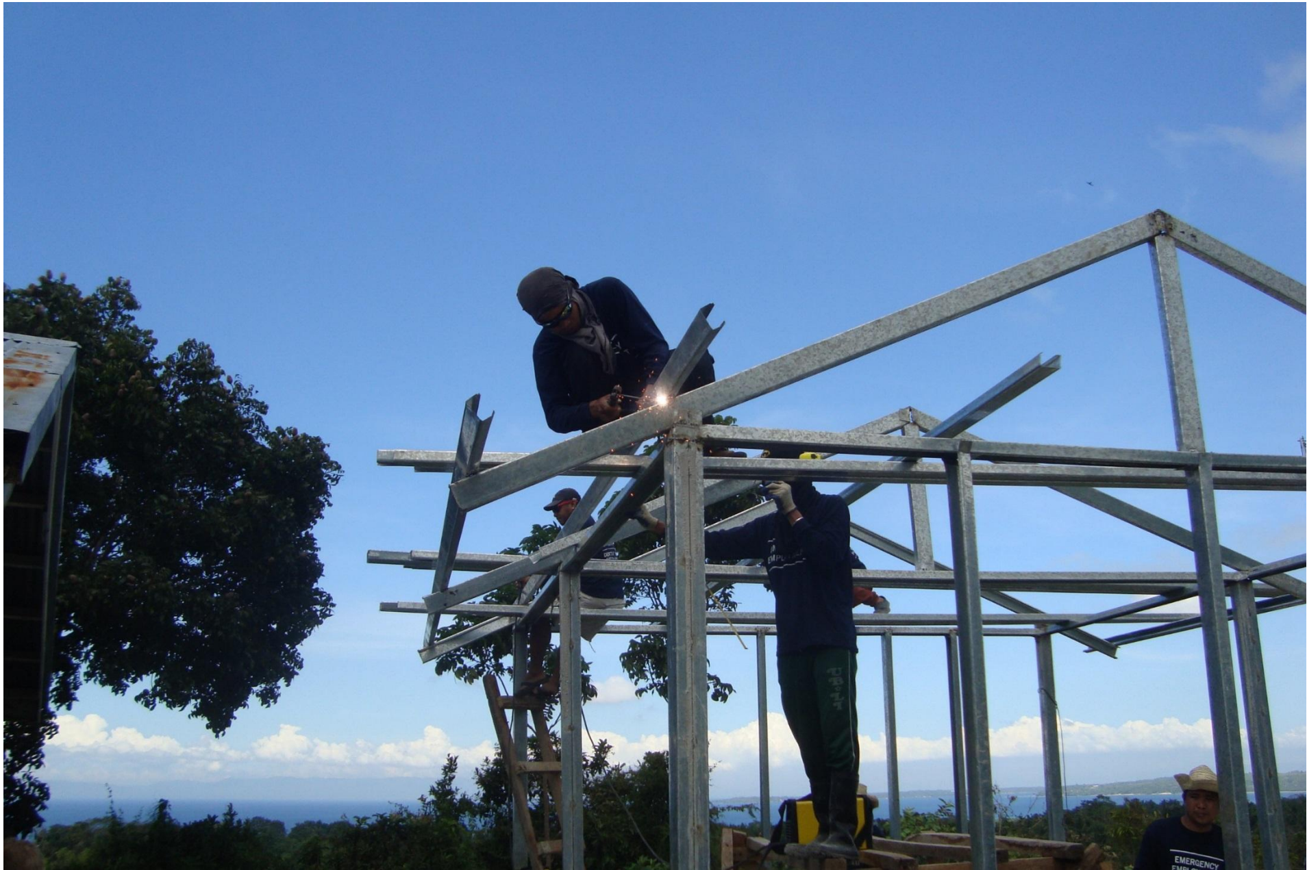
Trained on welding for the construction of permanent shelters.
