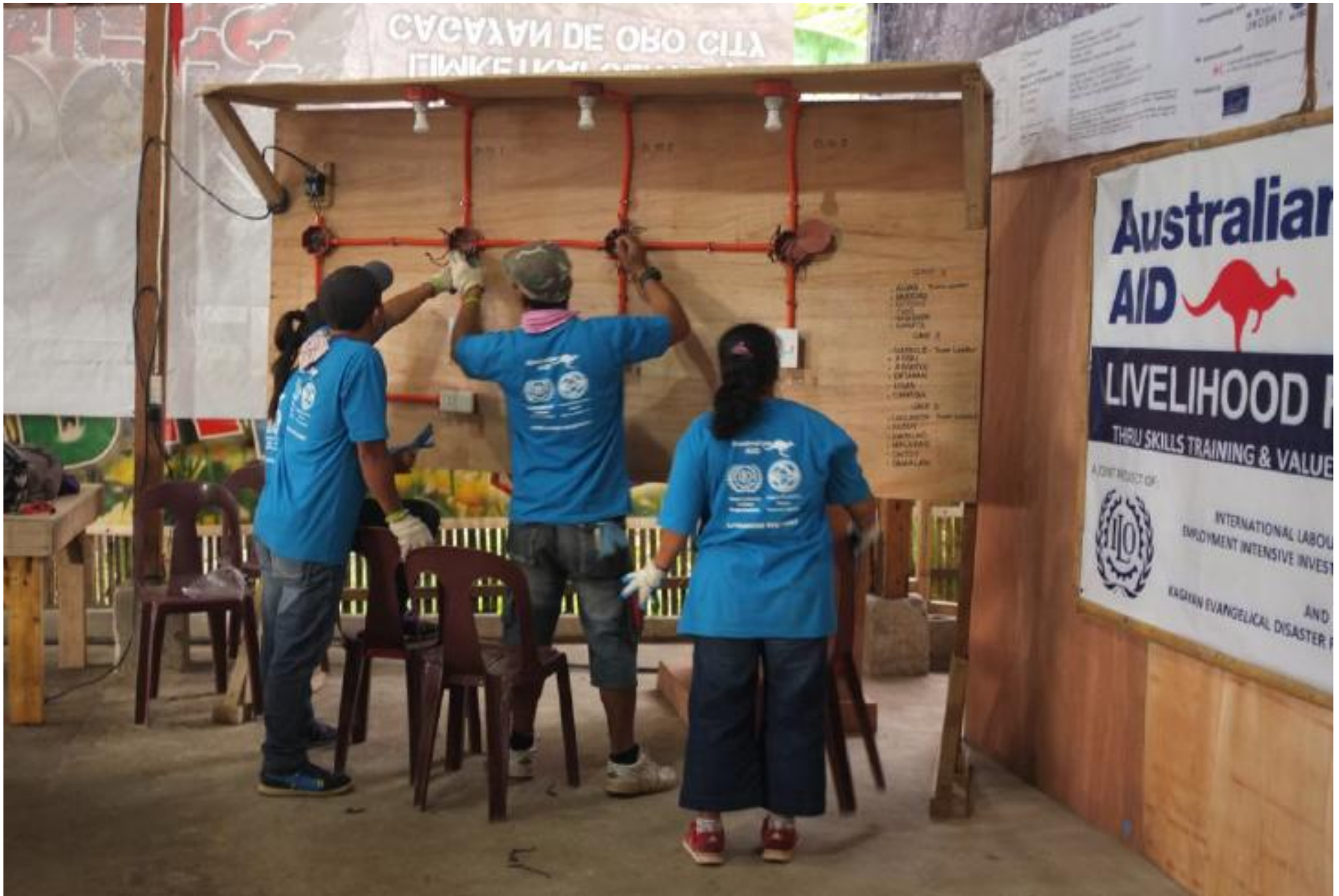
Trained on electricity installation for permanent shelters.
