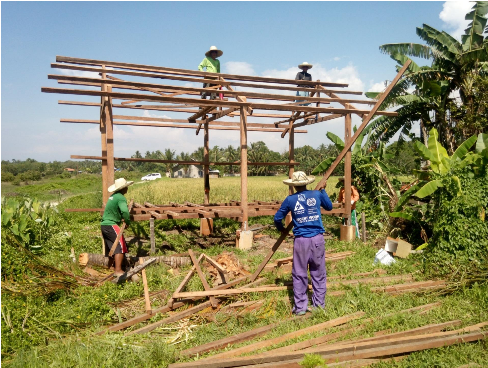
Assisted in the construction of semi-permanent shelter.
