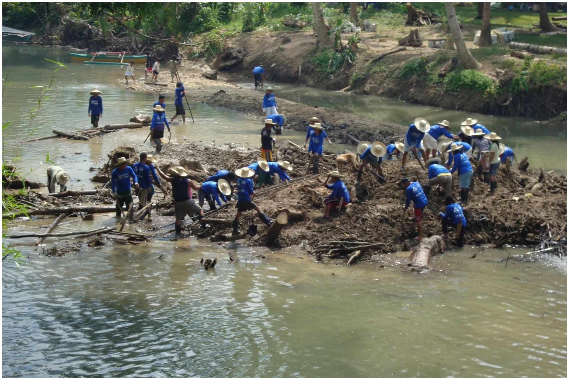
Local residents participated in removal and disposal of the debris.
